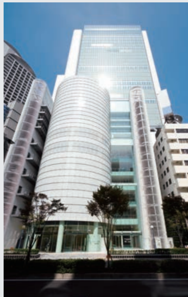
Completion: July 2008 Utility and function: Office, hall, retail/service establishment Total floor area: 84,749 m 2 Number of floors: B3F-34F and 1 penthouse floors
